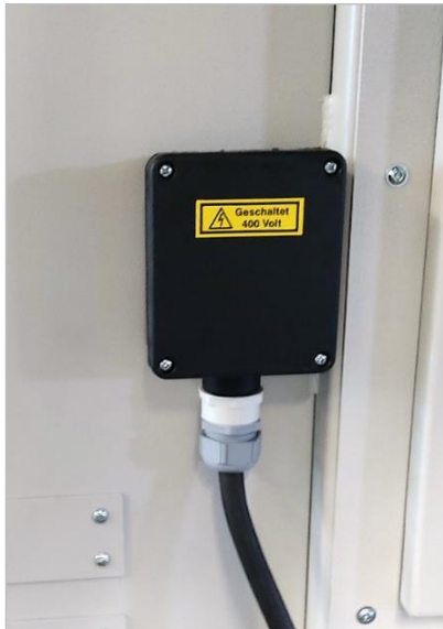
Figure 16: Electrical connection
